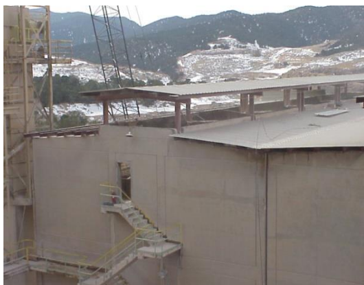
Figure C-3: former GCC baghouse, exterior
