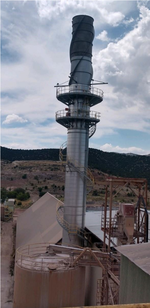
Figure C-1: GCC stack. A stack test is performed by inserting equipment through a "port" located at one of the circular observation decks visible on the stack.
